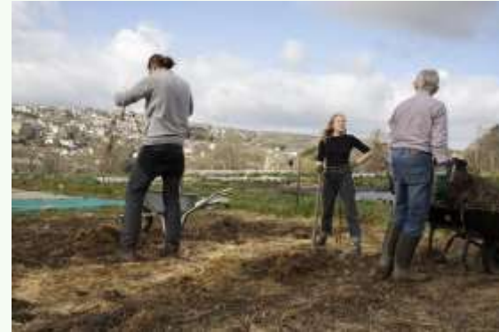
Volunteers preparing the ground
